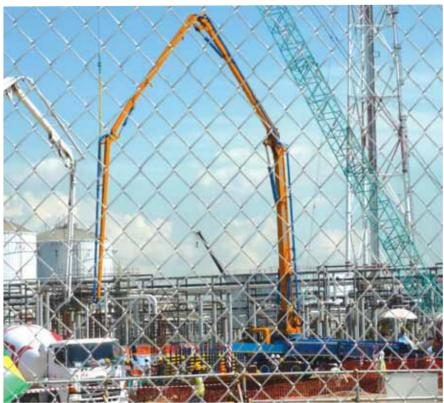
New 42m Boom Length Concrete Pump Used to cast concrete at petrochemical plant in Jurong Island.
